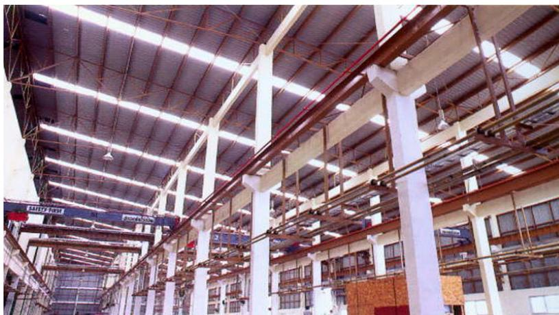
*Figure 5-1: Day lighting using polycarbonate sheets*
